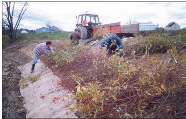
Photo 15: Installation de matelas de branches
